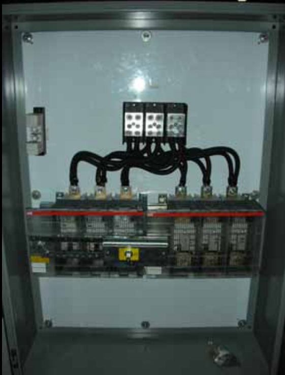
ABB Manual Transfer Switch 800 Amp Fused
